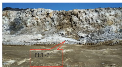
Figure 8: Exposed rock mass around chainage 380 m (PLT-7)
