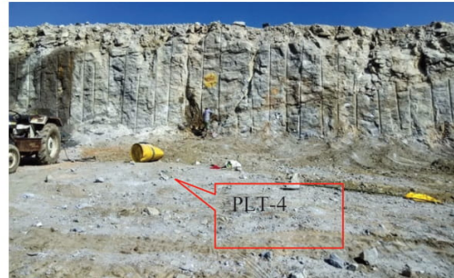
Figure 6: Exposed rock mass around chainage 310 m (PLT-4)
