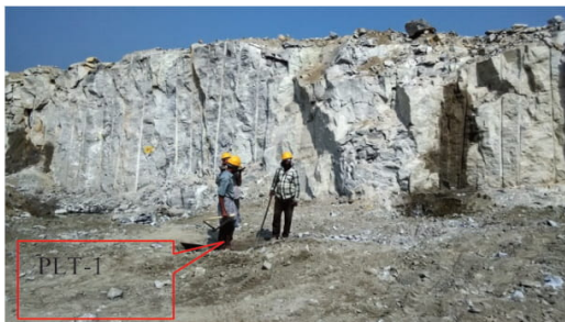
Figure 3: Exposed rock mass around chainage 60 m (PLT-1)
