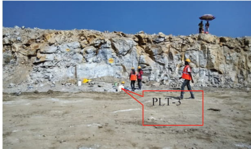
Figure 5: Exposed rock mass around chainage 200 m (PLT-3)
