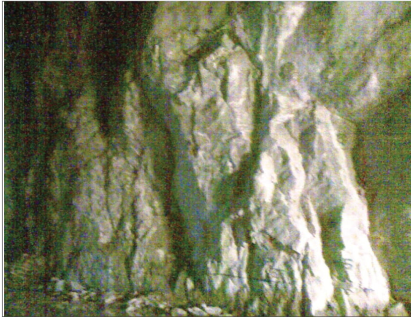
Figure 6: Shear seam SS4 on cavern walls
