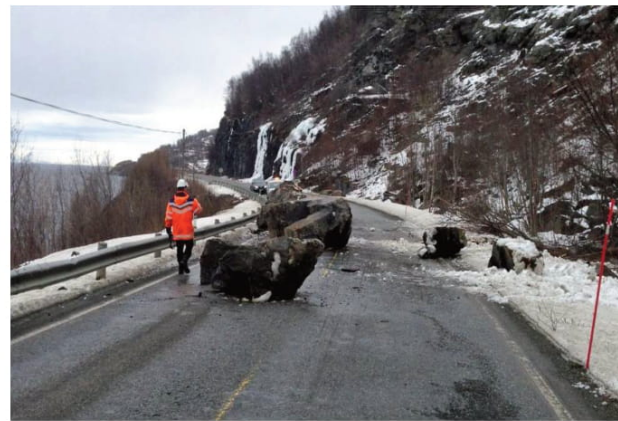
Fig. 12 - Nordnesfjellet in North Norway near Tromsø, Rock fall on the road (Tatensveivesen, Kåfjord commune)
