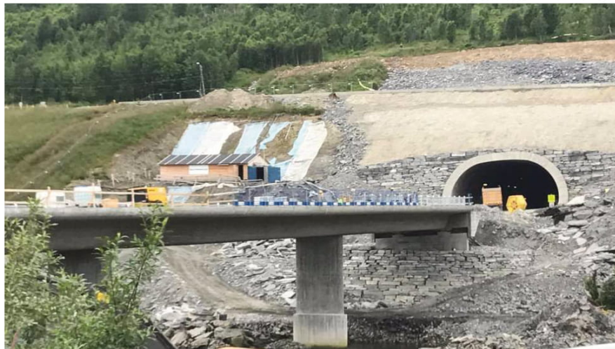
Fig. 13 - The entrance to Nordnestunnel from the Mandalen side (Photo: Jan Arild Hansen)
