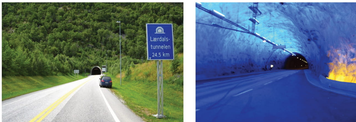
Fig. 9 - Entrance to Laerdal tunnel (left) and a safety cavern inside World's longest road tunnel (right)
