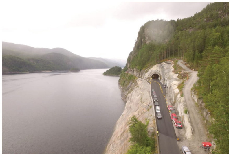
Fig. 10 - Bjorkaastunnel bypassing hazardous rock fall areas along the coast
