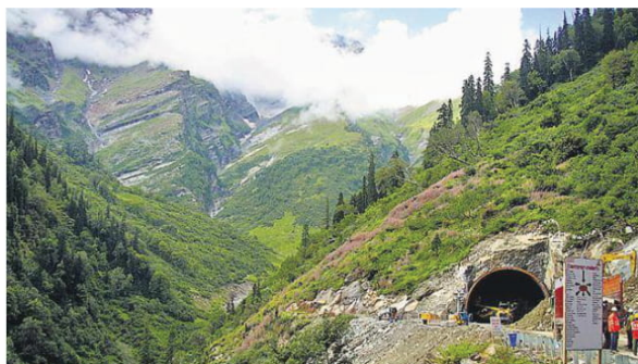
Fig. 2a - The southern portal at Rohtang Pass (HT photo)
