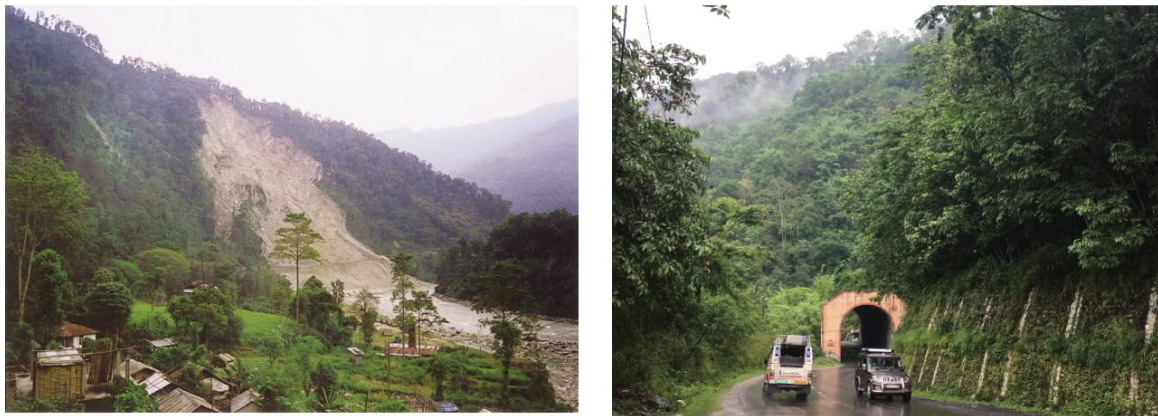
Figs. 7 a & b - The Burdang slide adjacent to the river Tista in Sikkim and the recent construction of a tunnel and retaining wall for mitigation of the landslide
