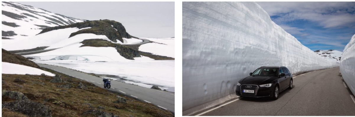
Fig. 8 - Photos showing the summer road above the Laerdal tunnel (commons.wikimedia.org/wiki)
