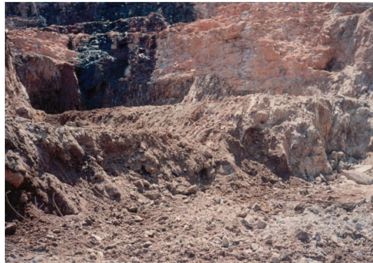
Fig.20: A general view of foundation rock mass at Bhadra dam
