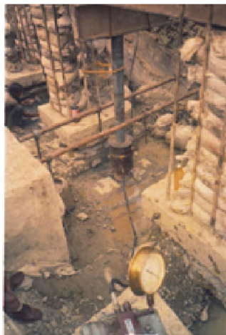
Fig. 1: Plate load test setup for deformation modulus with rigid plate method
