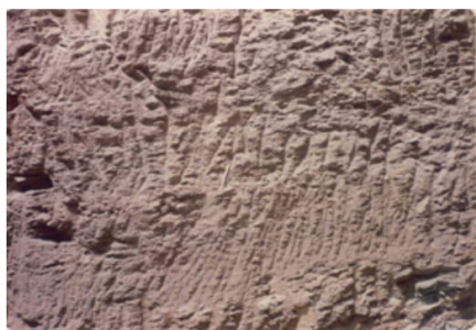
Fig.15: Weathered and disintegrated granite gneiss rock strata at EL 522m
