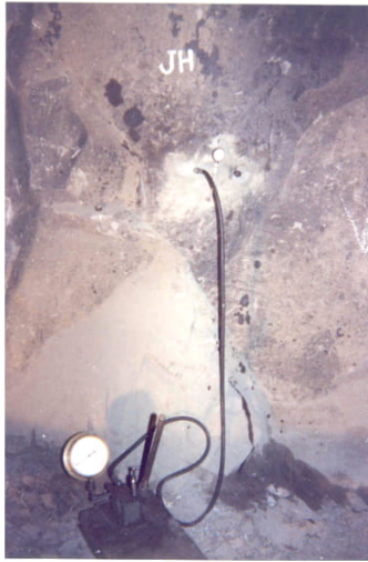
Fig.7 - Flat jack test in progress
