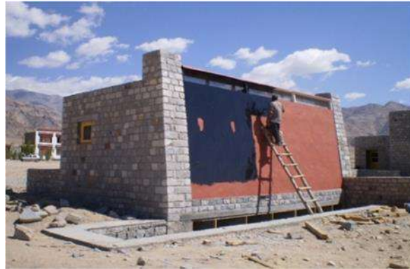
Figure 6 -Use of sun-dried earth blocks for construction (Nasir & Kamal, 2021)
