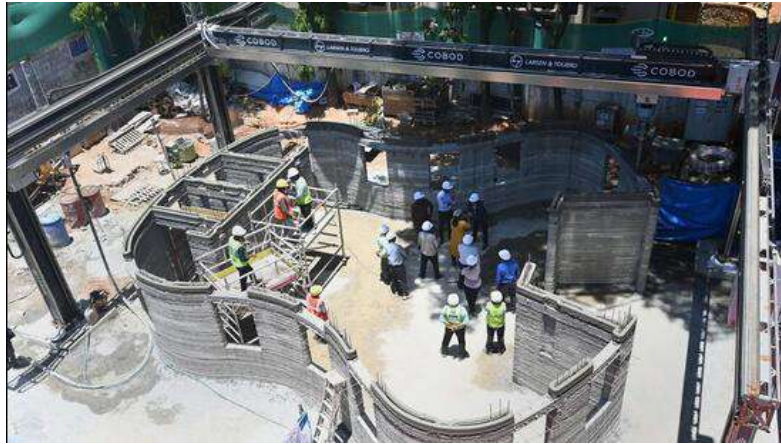
Figure 9 - A typical 3D printed construction
