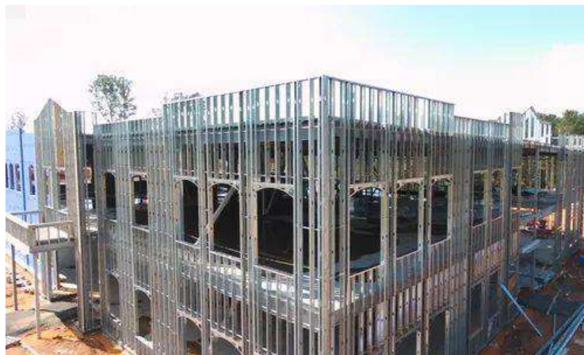
Figure 8 - Tubular steel light frame-based structure
