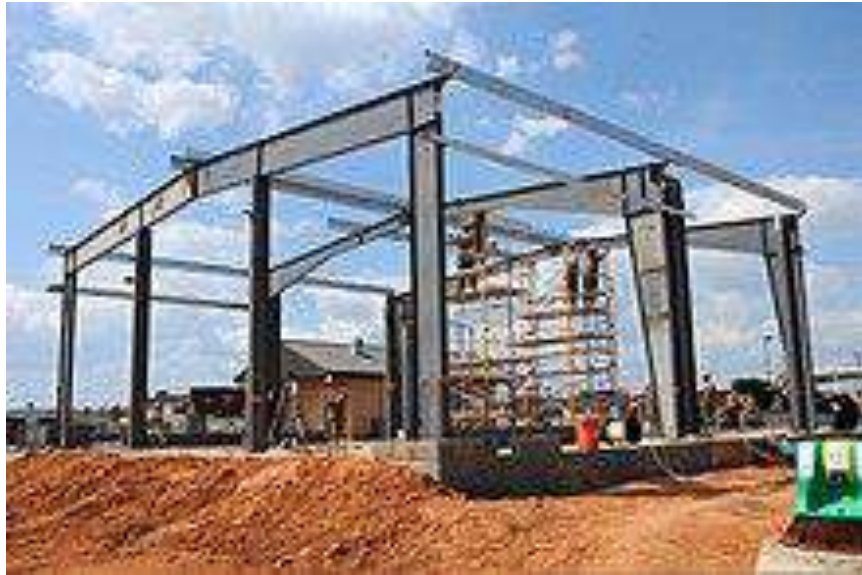
Figure 7 - Frame work of a pre-engineered building
