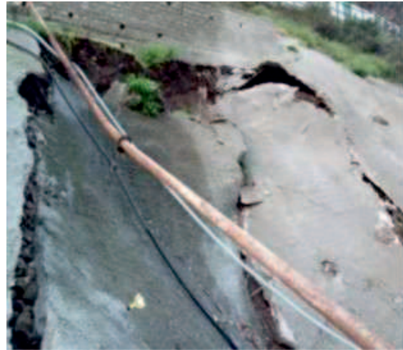
Figure 13 - Subsidence above tunnel
