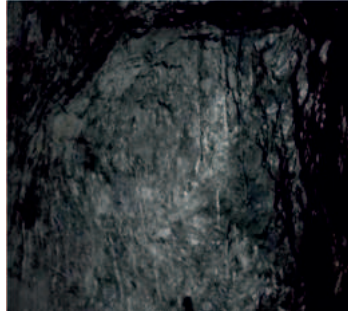
Figure 10 - Cavity at Ch. 257 m
