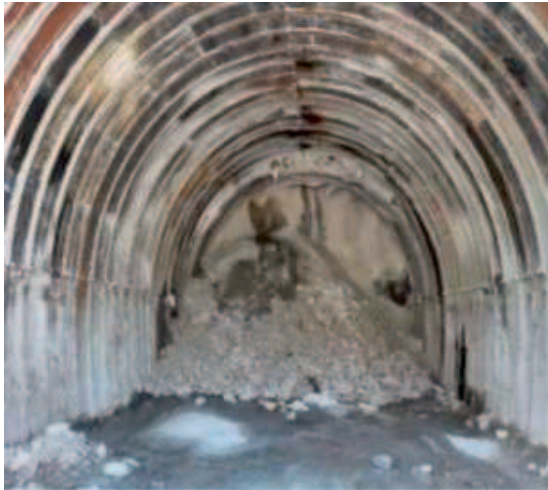
Figure 12 - Loose fall inside the tunnel
