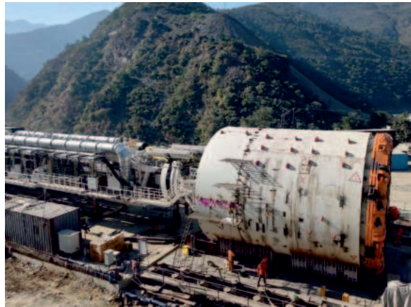
Figure 1 - Assembly of the single shield TBM at the Devprayag portal of the tunnel
