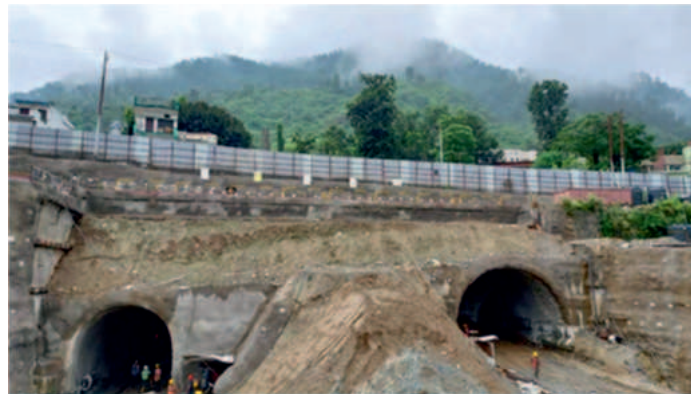
Figure 6 – Photograph of escape and main T11 at portal 1
