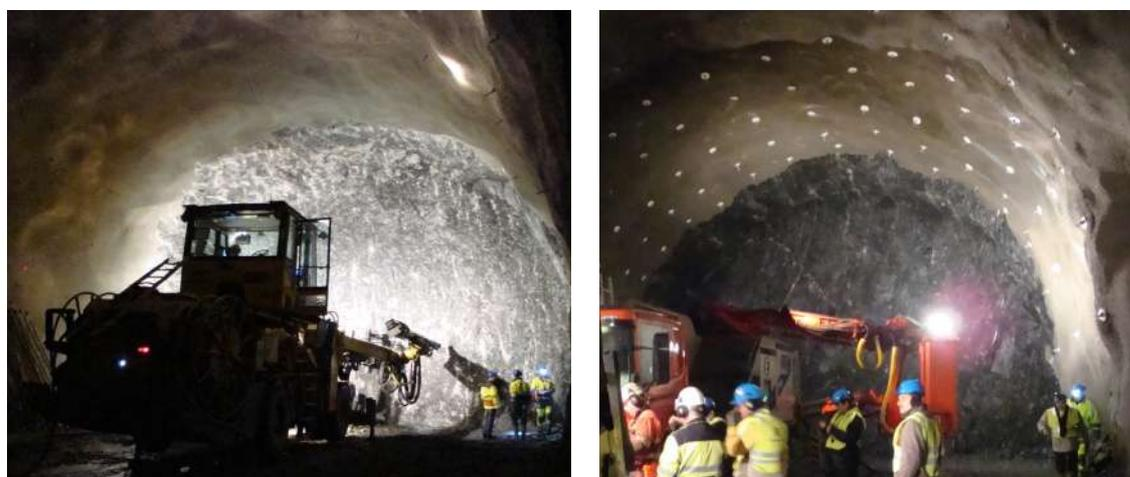
Fig.1 - Left: drilling next pre-injection screen. Right: preparing for primary robotic layer of S(fr), prior to bolting
