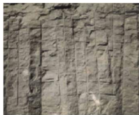
Fig. 24: Vertical joints at RAPP units 3 and 4
