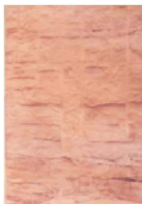
Fig. 23: Horizontal joints at RAPP units 3 and 4
