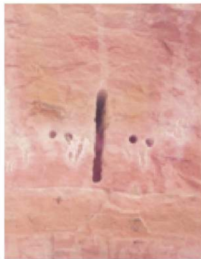
Fig.25: View of slot cut in the vertical direction at RAPP units 3 and 4
