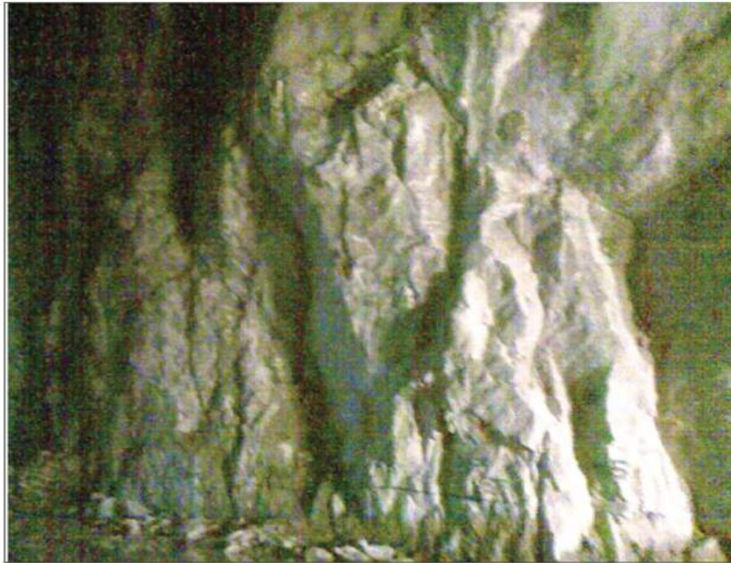
Figure 6: Shear seam SS4 on cavern walls
