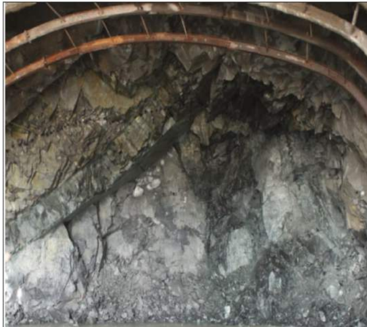
Figure 5: Dolerite dyke in access tunnel
