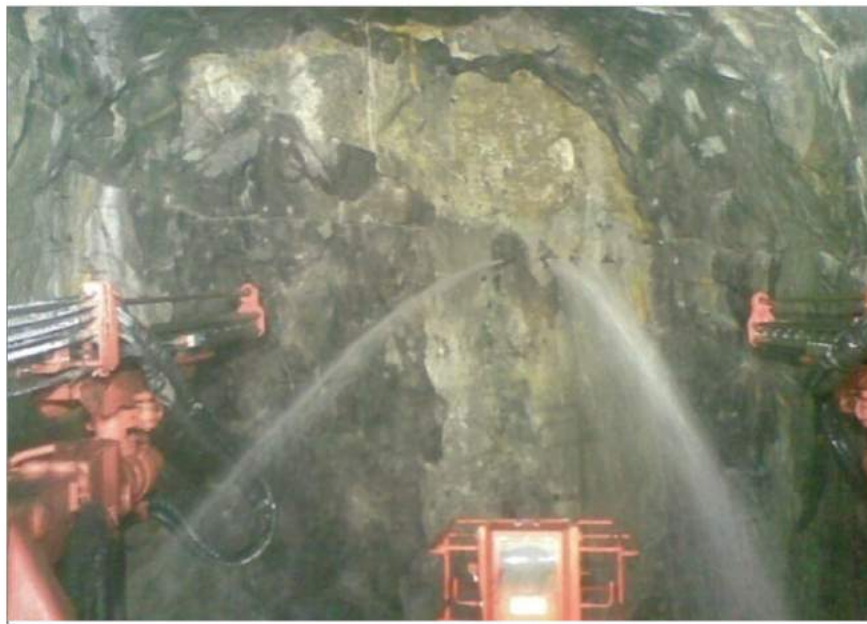
Figure 1: Water ingress during excavation
