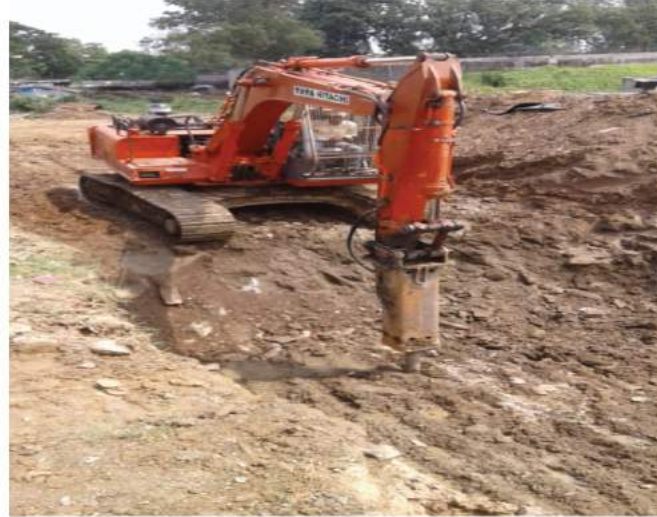
Figure 1: Rock cutting by breaker in progress at P4 site
